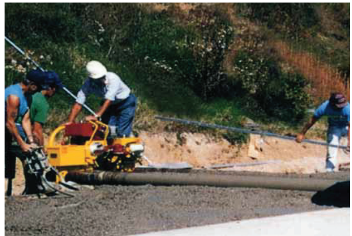
The Roller Screed does a great job on many types of concrete finishing such as roads, runways, bridges, inclines, etc.
