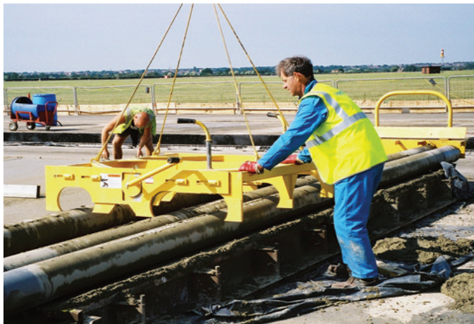
The lifting cradle makes transportation and setup efficient and simple.
